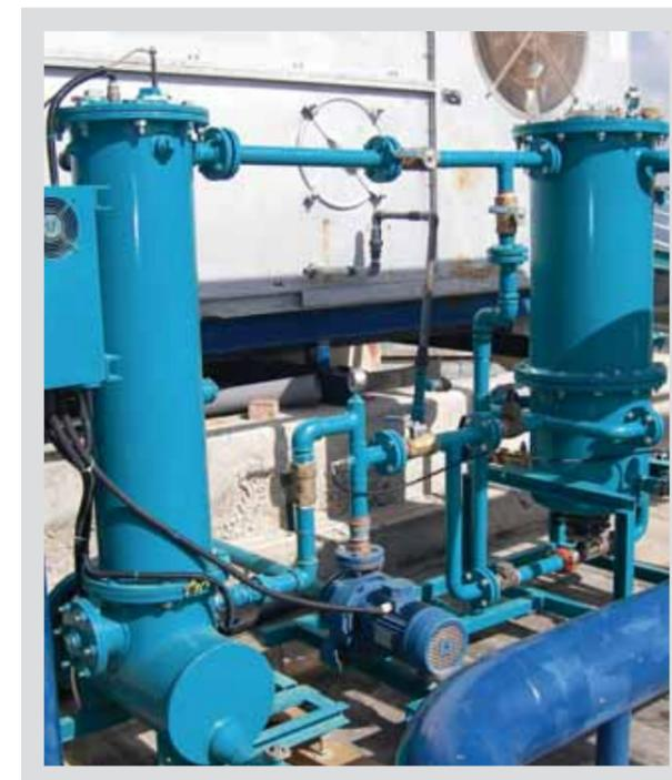
Installation of a Scale Remover model SR-05 with a Send Media Filter model SF-20-04.
