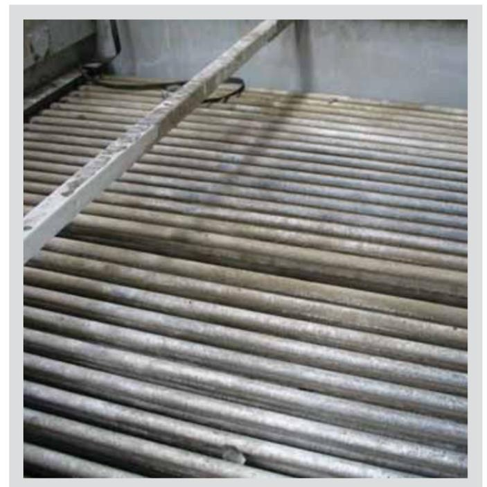
clean cooling tower after 3 years of using ball tech energy Scale Remover model SF-20-04.
